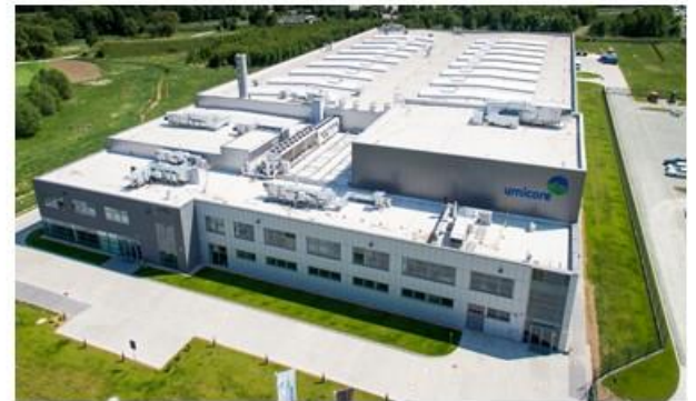
Nowa Ruda plant AC, Poland
