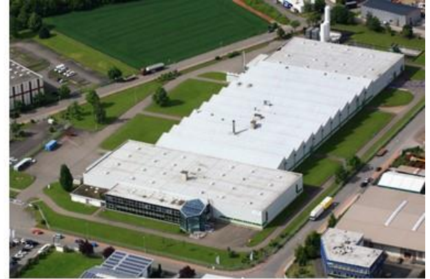
Bad-Säckingen plant AC, Germany
